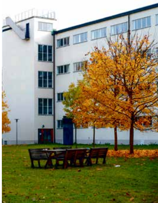
The Sveaplan building from behind.
